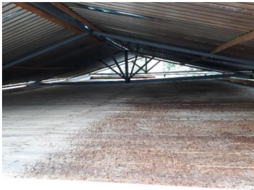
Figure 4.12: "Elba" or roof (on wheels) for drying the fermented cocoa beans. the rooftop is mobile, so it can protect the beans if it rains
