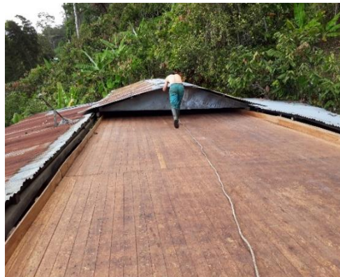
Figure 4.12: "Elba" or roof (on wheels) for drying the fermented cocoa beans. the rooftop is mobile, so it can protect the beans if it rains
